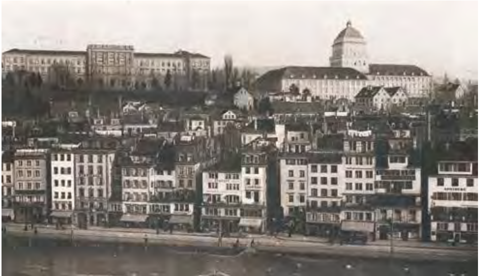
“Zurich – old and new university”: In 1914 the University of Zurich moved from the south wing of the Semper building to its new facility. Contemporary postcard.
