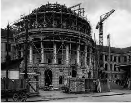
Renovation and expansion of the main building according to Gustav Gull's design. Central block of the new east façade with rotunda and cupola, ca. 1919.
