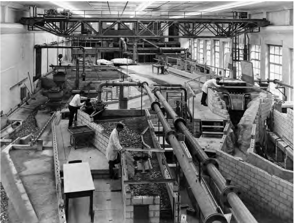
Above: Glass demonstration tank in a lecture hall of the Experimental Station for Hydraulic Engineering, 1930.
