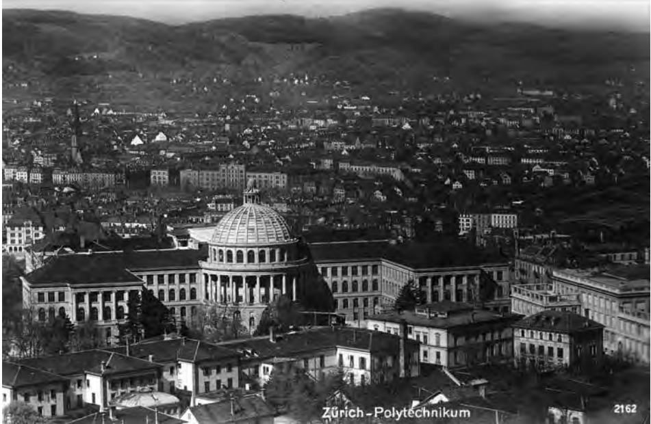
The prefabricated reinforced concrete structures of the cupola were later covered with tiles. View of the east façade, 1920.
